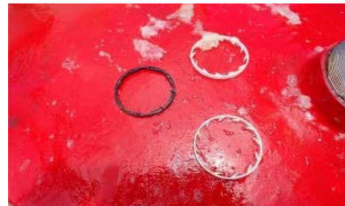
Figure 2. Internal inspection of the foam tank for a helideck foam system (above, left). In this particular instance, 60% of the foam was found to be in a gelatinous state after different types of foam had been mixed, rendering the system inoperable. The locking caps from the cans were found floating inside the tank (above, right).
