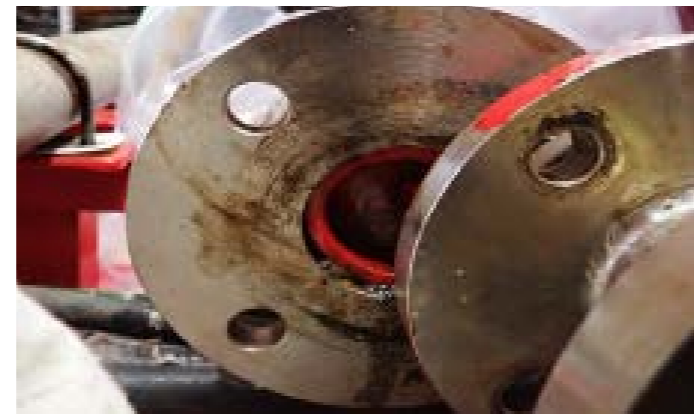
Figure 1. A protective cap (above, left) retrieved from inside a high expansion foam firefighting system (above, right), where it was restricting the flow of foam to the proportioner.
